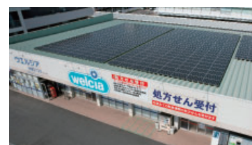
Store outfitted with solar panels
