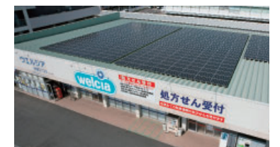
Store outfitted with solar panels
